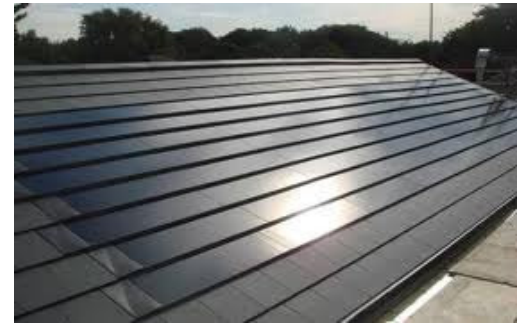
Figure 2. Aesthetic PV tiles for rooftop solar power generation
